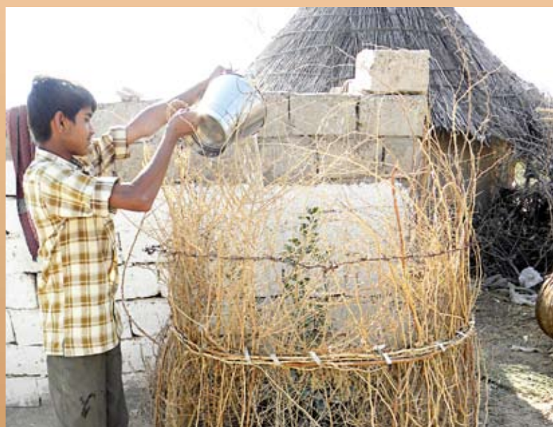
House hold soak pit for liquid waste management
